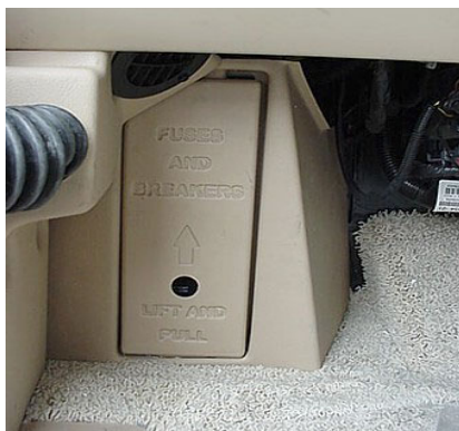
Automotive 12-Volt Circuit Breakers and Fuses (Located beneath left end of dash) -Typical View
