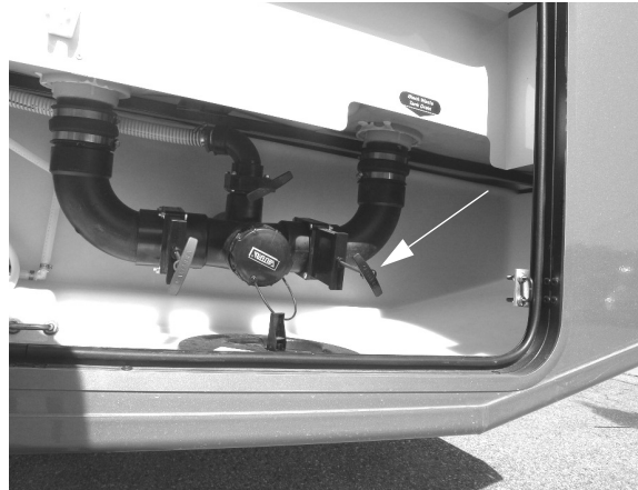
Black Waste Tank Drain Valve (Rear) (Located in water service center) -Typical View
